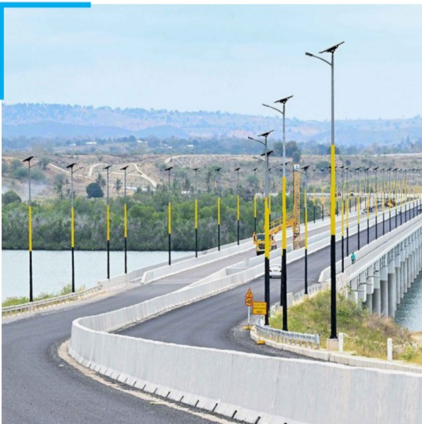
A section of Dongo Kundu Bypass road that was recently launched
